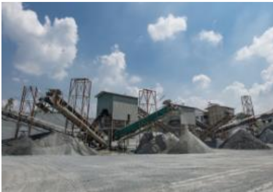
Figure 22: Tongkah Harbour activities for andesite extraction are concentrated in the Saraburi province
