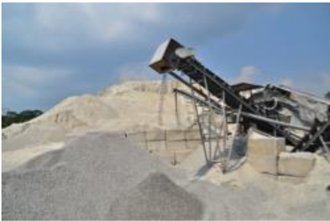
Figure 6: Soon Yong Huat Recycled Concrete Processing Facilities
