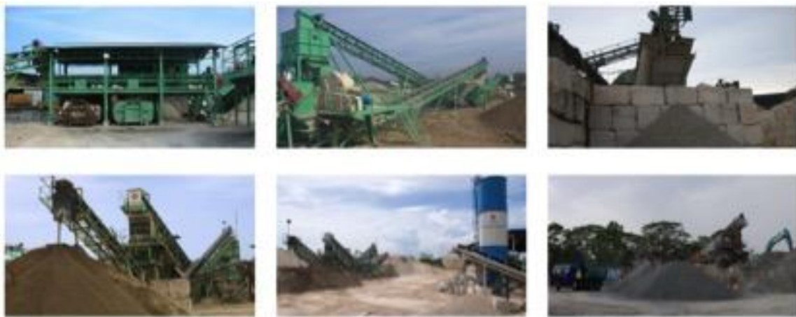
Figure 4: SamGreen material Recycling Facilities Source: Samwoh
