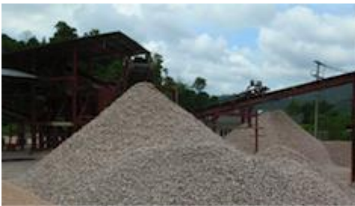
Figure 18: Inthai Crushing Plant
